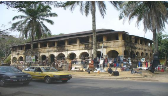
Figure 6: Old German building in Dja (Villa Mandessi Bell)
