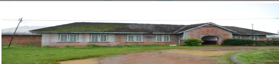
Figure 7: ENIEG Kumba Administrative Building
